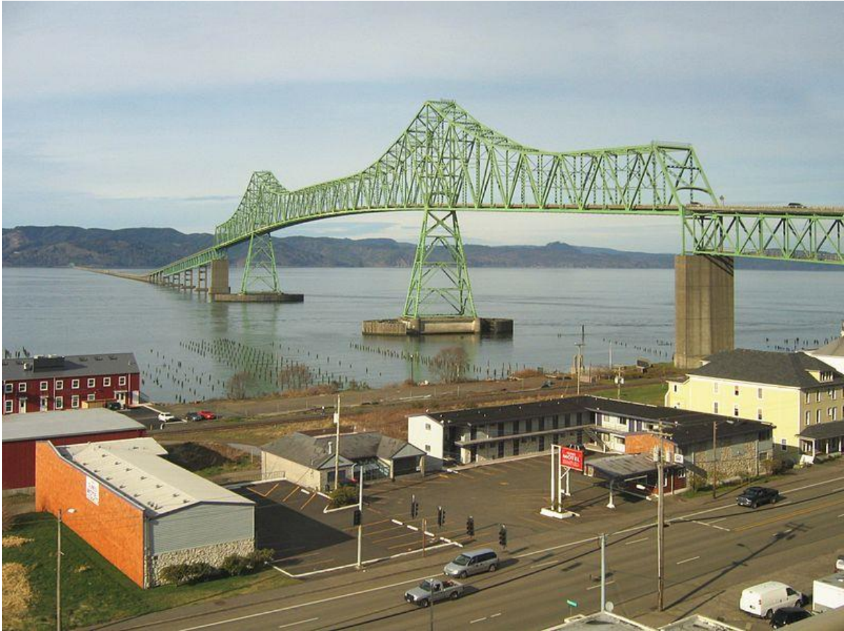
Figure 3 Photo of the Astoria-Megler Bridge from the South ramp. Architectural projection made with hugin. (2008). Wikipedia. https://commons.wikimedia.org/wiki/File:Astoria-Megler_Bridge01_2008-02-26.jpg
